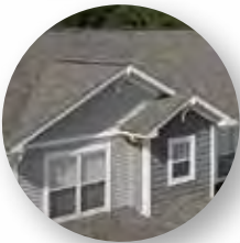
Roofing and Ventilation
